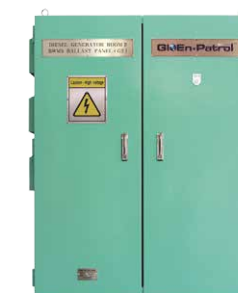
UV Power Supply Panel
