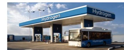
Hydrogen filling stations
