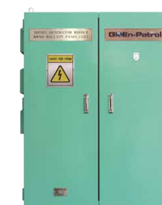
UV Power Supply Panel
